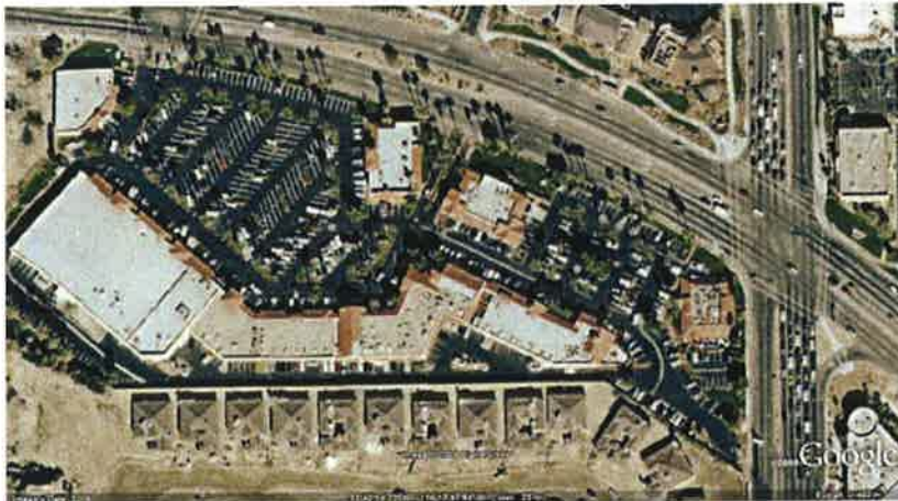
This is the SW Corner of Washington Street and Route 111. Note the lack of connection between the commercial activities and the homes located immediately adjacent to the center.
