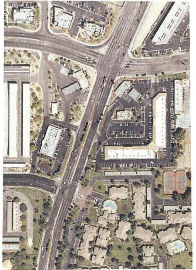
Deceleration Lanes Northbound at Shopping Center & Southbound at Shopping Center South of Country Club Drive
