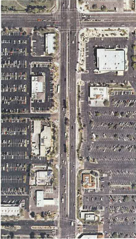
Deceleration Lanes Northbound at Ralph's Shopping Center & Southbound at Albertson's Shopping Center South of 42 nd Avenue
