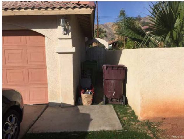
Trash container storage and debris
