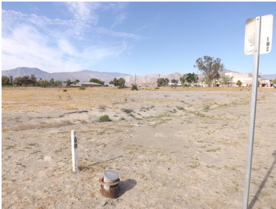
Photograph 8. Southerly view from Westward Ho Drive, including water infrastructure.
