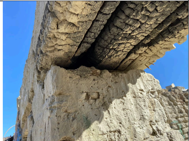
Representative view of crevice habitat suitable for day-roosting bats and maternity colonies at the abandoned adobe.
