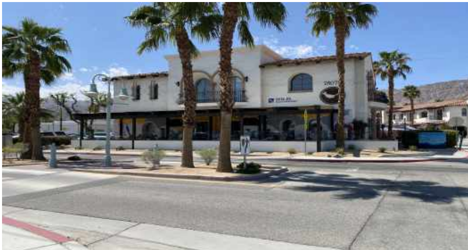
Above: RD RNNR Outdoor Patio Modification by Applicant
