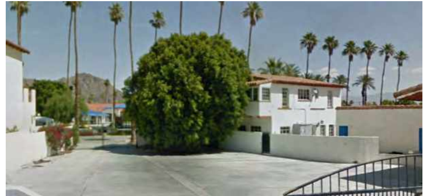
EXISTING CONDITION OF SITE OF FUTURE OASIS - BETWEEN MUSEUM AND LUMBERYARD
