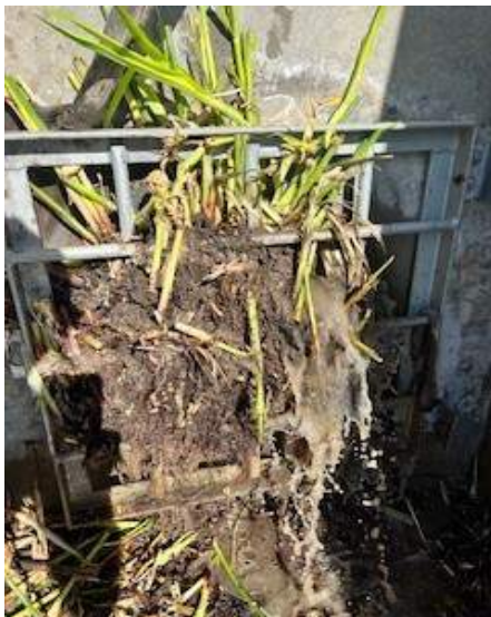
Storm Drain Maintenance - Before
