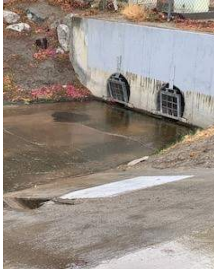
Storm Drain Maintenance - After
