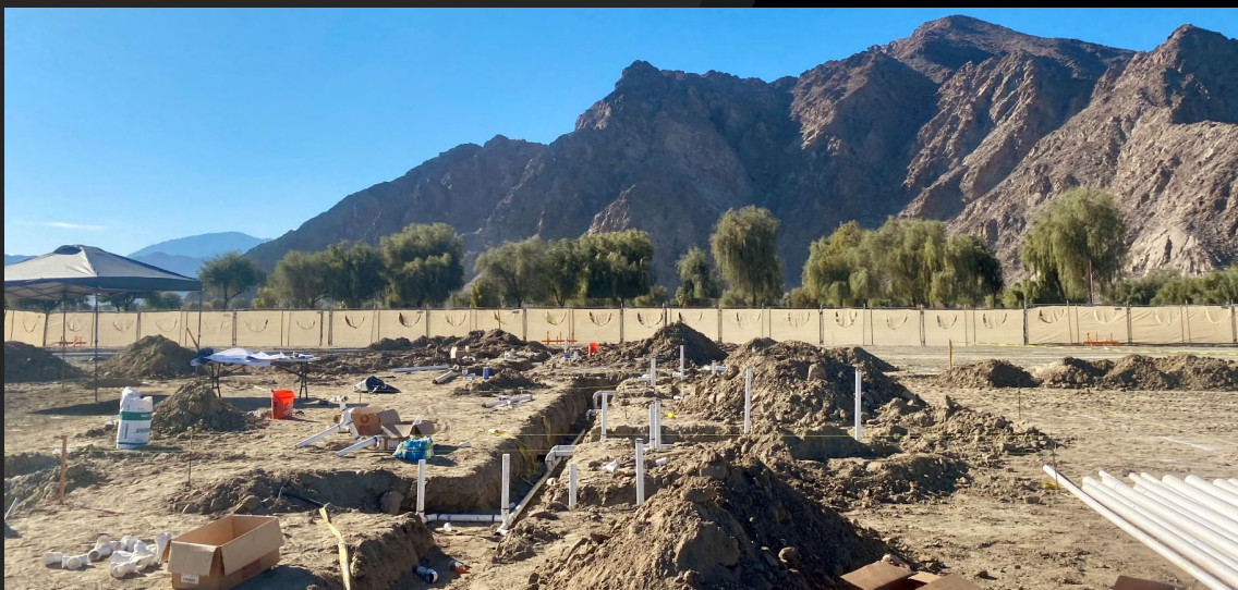
Progress Photo – Conference and Shared Services Building
