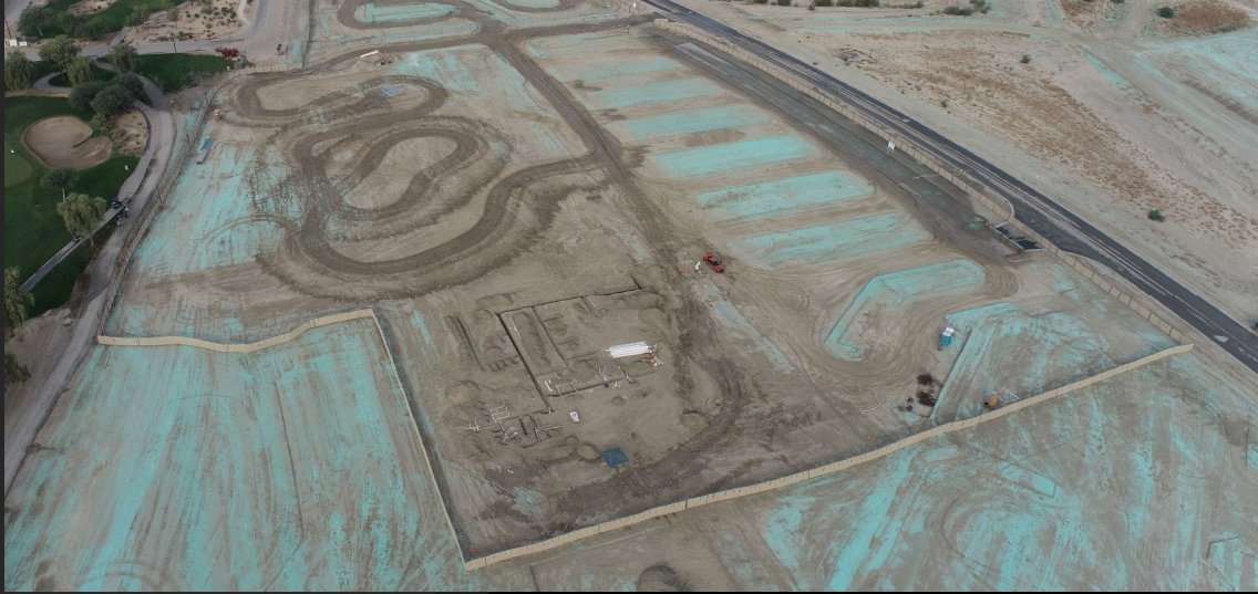
Progress Photo – Conference and Shared Services Building
