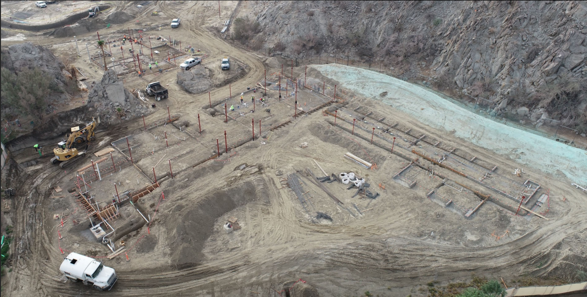
Progress Photo – Montage Spa
