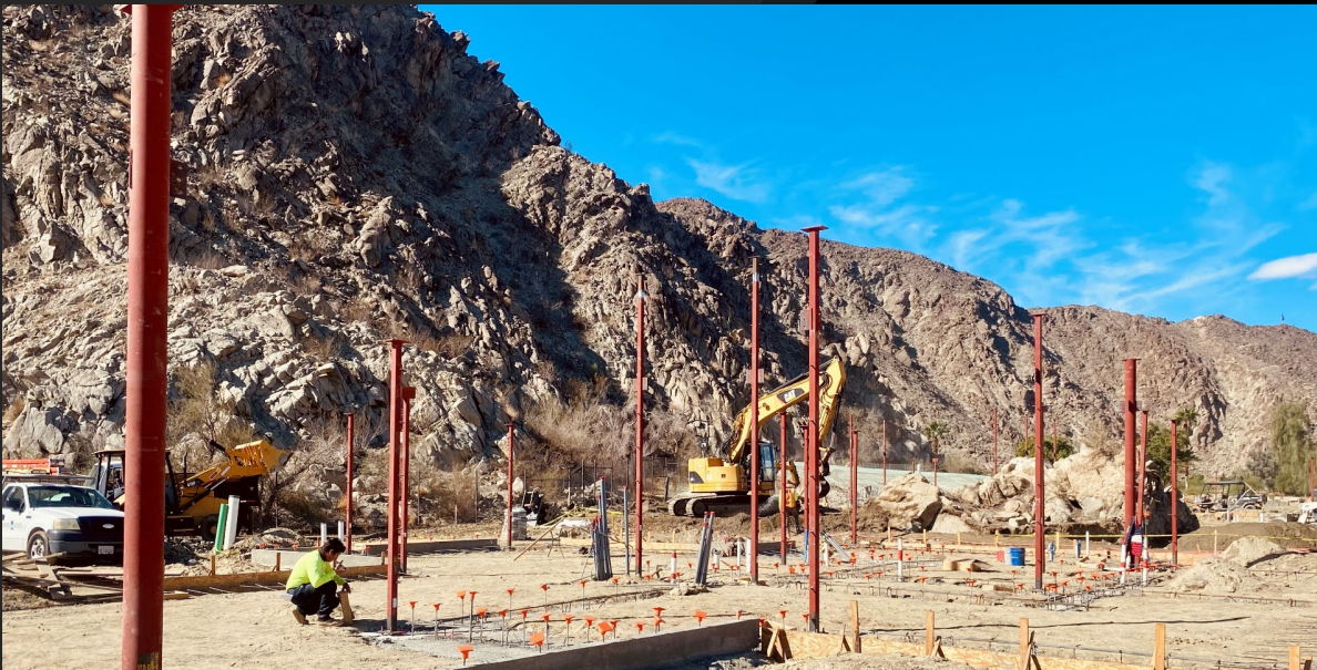
Progress Photo – Montage Spa
